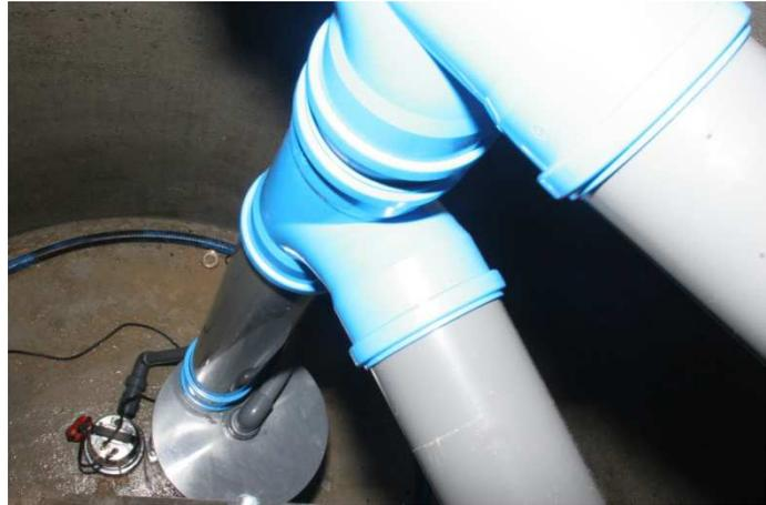
18. Check all connections and screw unions. The tank inlet is connected to the tank outlet and has a downward gradient of at least 1% (3% is desirable) towards the outlet. From this line, a second line leads vertically downwards into a DN 100 branch, which leads directly to the DN 100 inlet connection on the filter unit (C). A hose is attached to the screw connection on the filter unit (C) and leads directly to the flushing pump (D).
